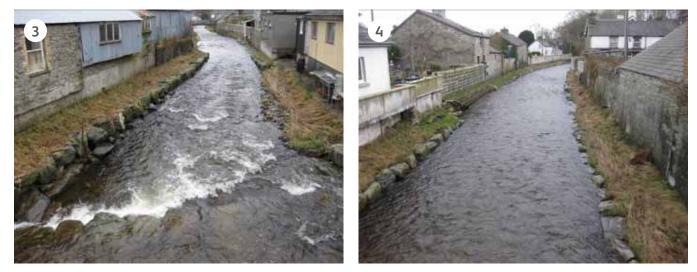
(3) Rock and geotextile revetments and a blockstone check structure at the upstream end of the regraded reach; (4) Rock and geotextile revetments on both sides of the channel.
