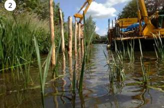
Survey line for position of retaining posts for coir rolls.
