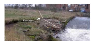
A 1.8 m wide Larinier Superactive baffle fish pass was constructed to enable fish passage over Heatley Weir, requiring two flights with an intermediate resting pool. The fish pass was located immediately below the weir on the right bank, and the fish pass routed
