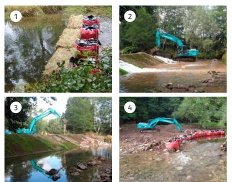
(1) Straw bales in place as a downstream sediment trap;
