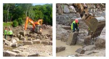
(1) View downstream during construction;(2) Installing tombstones to low stone weirs
