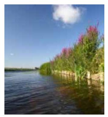
An eroded and undercut bank exposing bare earth at the water margin was restored using coir rolls pre-established with native water plants to create a naturally regenerating revetment and to restore water vole habitat.
