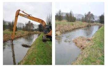
Construction of deflectors using dredged material
