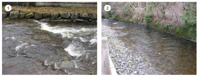
(1) Blockstone check structure preventing upstream erosion, (2) Bar forming on right-hand bank.
