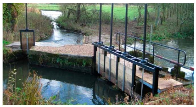
Hyford Hatches: restored allowing more effective and safe water level management through operation control. All images © Environment Agency copyright and database rights 2013
