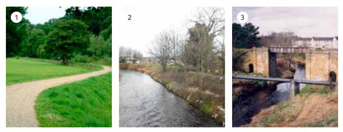
(1) Existing flood embankment to be breached, with set back embankment constructed behind; (2) Flood plain to be lowered behind embankment shown here, with set back embankments constructed and buildings removed; (3) Bridge to be removed.
