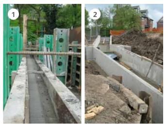
Concrete U-channel of the fish pass during construction;
