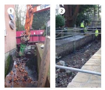
(1) Lowering of the existing weir; (2) Installing gabion baskets in dry-working area behind clay-bunds
