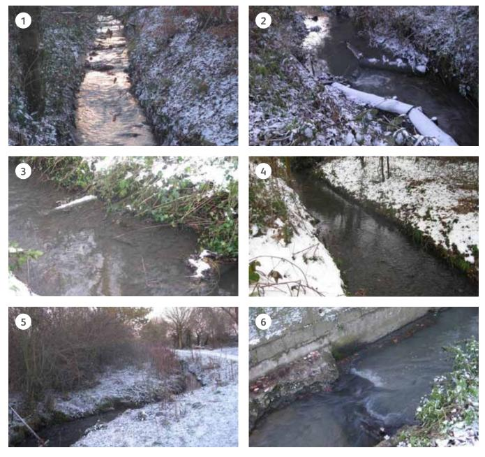
(1) Reach where toe-boarding has been removed; (2) pine-box deflectors backfilled with gravel; (3) small flow deflectors; (4) artificial riffle in a straightened section of the channel; (5) remeandering of previously straightened channel; (6) former location of weir with concrete base and banks retained.
