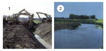
(1) Relocation of IDB drain and flood bank set-back;(2) Removal of flood bank and marginal berm creation.
