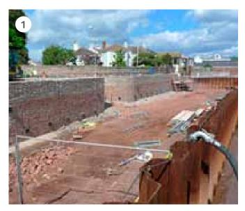
(1) Construction of two walls of the Shaldon and Ringmore tidal defence scheme, into which ecological enhancements were incorporated. May 2010 All photos © Larissa Naylor copyright and database rights 2013
